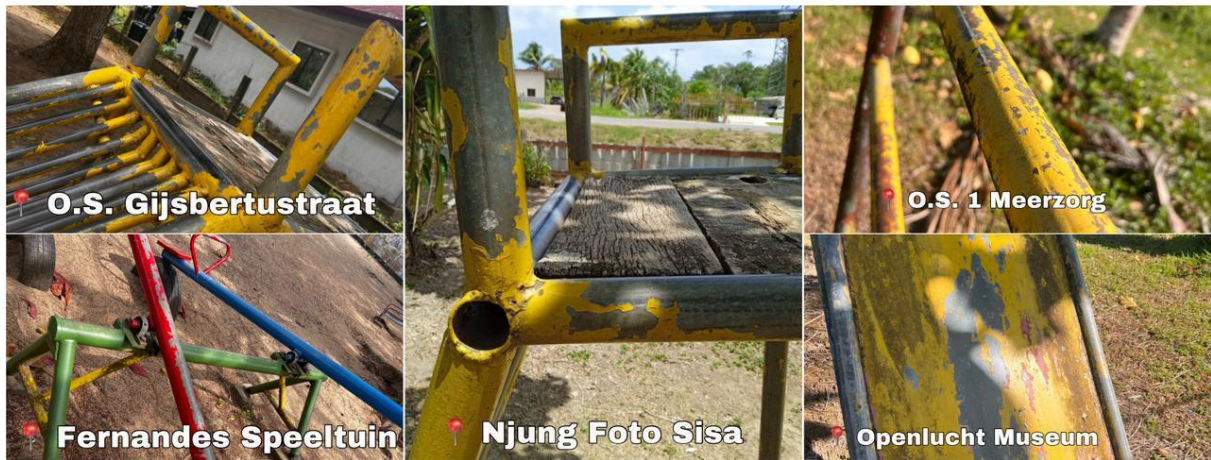
Figure 5 Overview of the flaking paint on the equipment at five different locations
