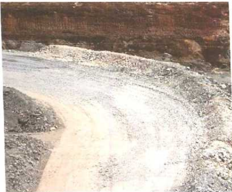
Figure 2.7: Haul road, capped with crushed rock ( RGM)
