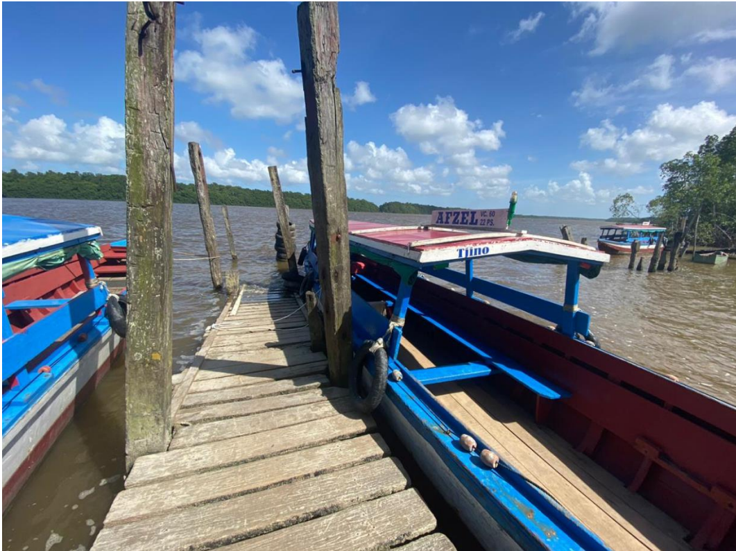
Figure 4.4 Scaffold at Mon Trésor
